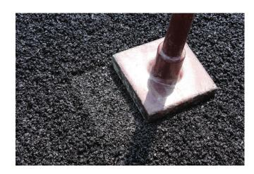
Ideal for the repair of potholes and other defects in bituminous and cementitious surfaces especially in wet conditions and on heavily trafficked roads.
