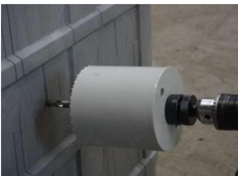
Drilling hole for cable entry
