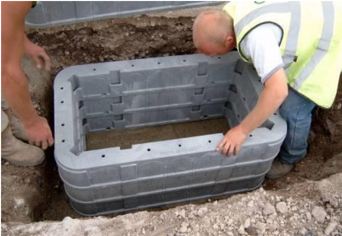
Stacking sections to form chamber.
