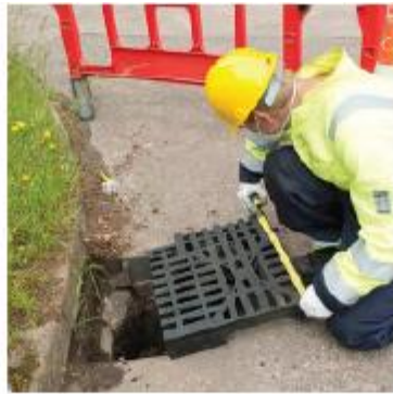
Measure MultiGrate and mark up for cutting using the moulded lines as a guide.
