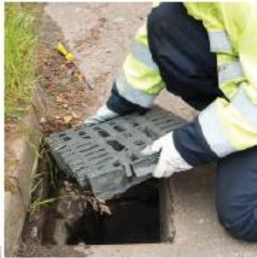
Check fit and adjust where needed. Note that the grate can easily be handled by one person.
