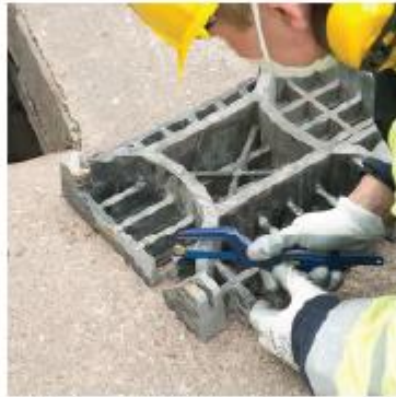
Adjust the grate to fit internal intrusions of the existing frame by using a small hand saw.
