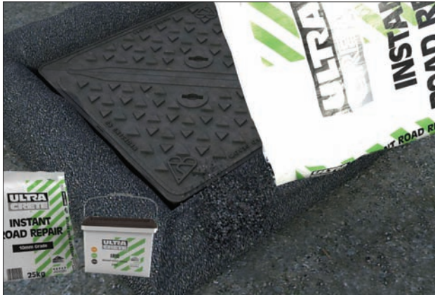
Figure 7 Installation of Ultracrete Instant Road Repair
