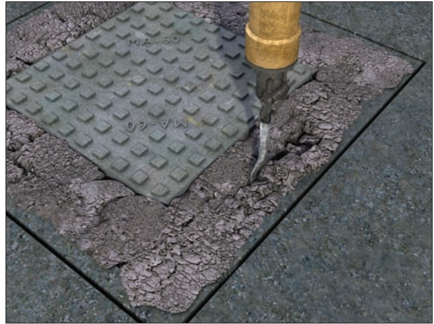
Figure 2 Excavating failed ironwork
