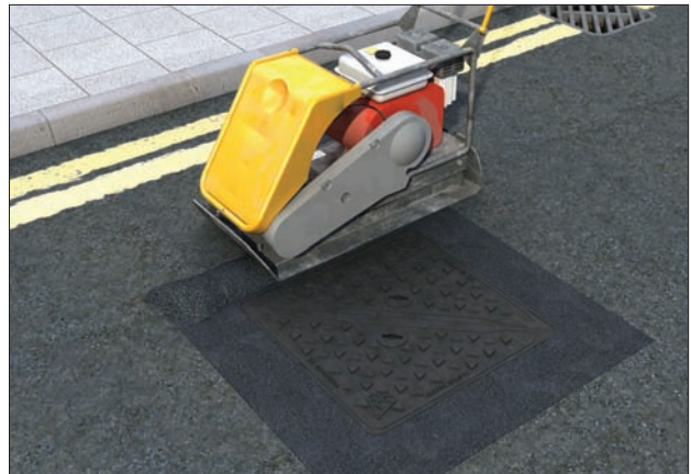
Figure 8 Final compaction of Ultracrete Instant Road Repair
