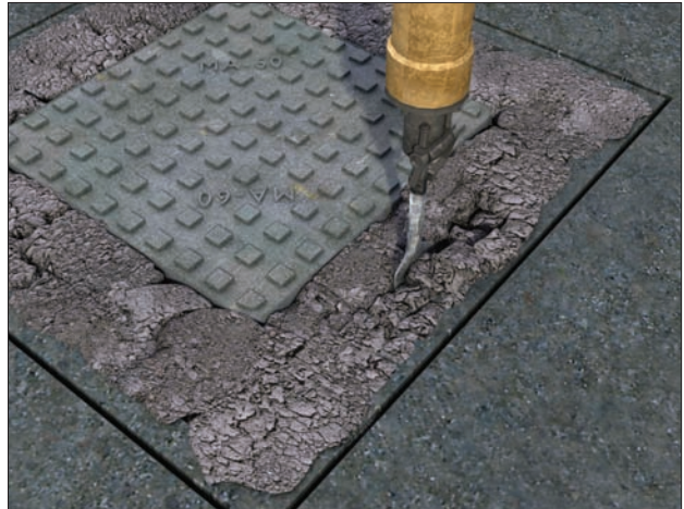
Figure 2 Excavating failed ironwork
