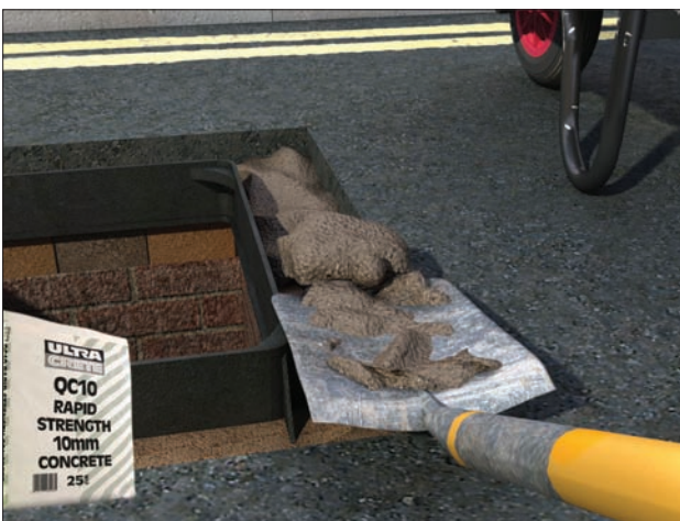
Figure 5 Backfilling using Ultracrete QC10
