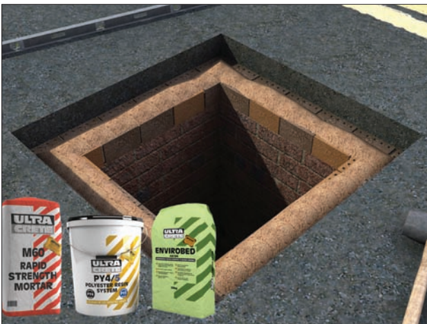
Figure 3 Apply the bedding mortar to the prepared substrate
