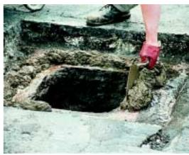
A rapid strength bedding mortar designed for the fast installation of street ironwork. Once applied, the road can be open to traffic after 90 minutes.
