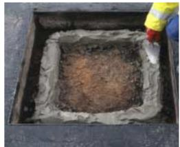
The market leading rapid strength bedding mortar designed for the fast installation of street ironwork from temperatures as low as +1°C. Once applied, the road can be open to traffic after only 60 minutes.
