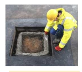
A cementitious bedding & repair mortar designed for the fast levelling of street ironwork
