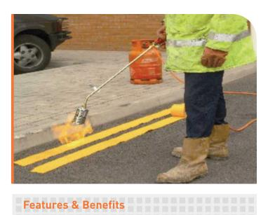
Ultracrete Instaline is simply cut from the roll and heated onto the road, Instaline offers all the qualities of hot applied thermoplastic with the benefit of an application time of just minutes.
