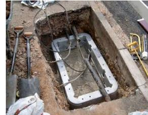
Set the first segment level on the base, bedding it firmly in, and check that it is level. The segment should be tamped into the base to provide a solid foundation for the chamber.
