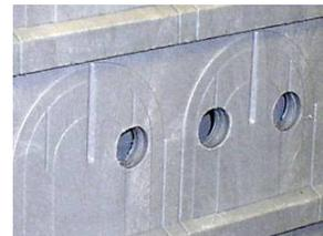
Note the secondary centre marks for positioning an array of smaller ducts
