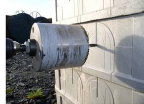
QUADBOX is marked with duct positions that ensure correct duct spacing and accurately aligned holes. Locate the pilot drill in the centre mark and drill at moderate speed so as not to generate excessive heat. Drill through both walls or, for precision alignment, drill separately from the inside and the outside using the drill centre marks.
