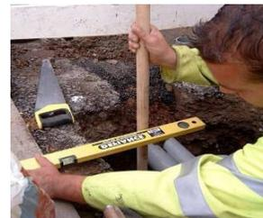
Install the additional segments of the chamber (with due allowance for the frame and cover installation) to the final depth ensuring that each layer is fully seated.
