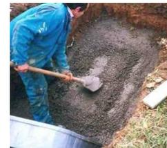
The floor shall be finished using a float and trowel to achieve an even surface sloped slightly towards the sump hole grating where the customer has specified a sump.
