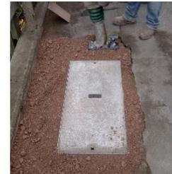
During the initial compaction around the chamber base, it is particularly important to avoid over compaction or ramming the side of the chamber to the extent that it might disturb its position.
