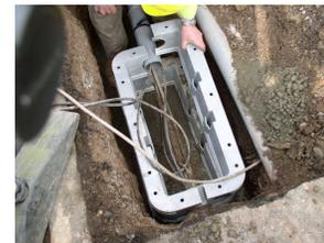
Alternatively, a ring may be drilled and then cut longitudinally for reassembly around an existing duct. In these instances, it is important that a complete ring is installed above the cut ring.
