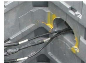
To build over existing cables or ducts, cut a suitably sized duct entry, see 'Duct Entries' section; then with a hand saw cut from the bottom of the ring to make an open bottomed arch.
