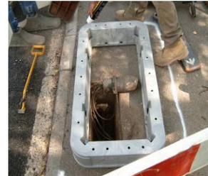
Within the marked area, excavate from the lowest point of the footpath surface to the total depth of the chamber. Allow additional depth for the concrete base and for the frame & cover. For a 5-ring chamber the excavation depth is 965mm. Additional excavation is required local to the sump.
