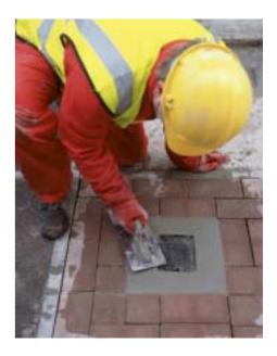
The market leading non-shrink concrete designed for reinstatements of ironworks and access covers on roads & pathways. The speed of application and ultra quick setting time reduces the risk of damage to the newly reinstated area.
