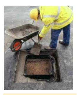
This market leading rapid strength concrete is designed for thick section concrete repairs and is an ideal system for backfill of carriageway ironwork.
